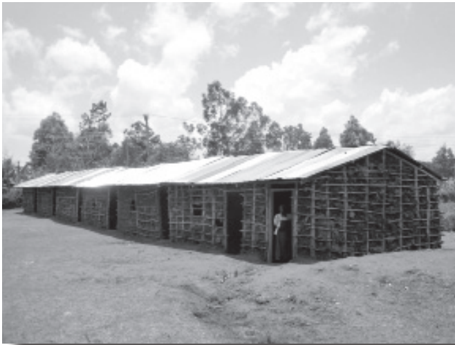
The new school at Emasara
